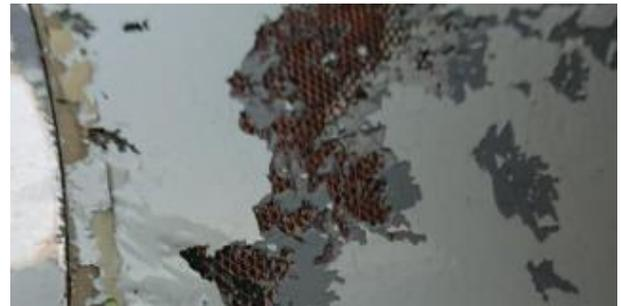
Fig. 4. Metal expanded mesh - damaged.
